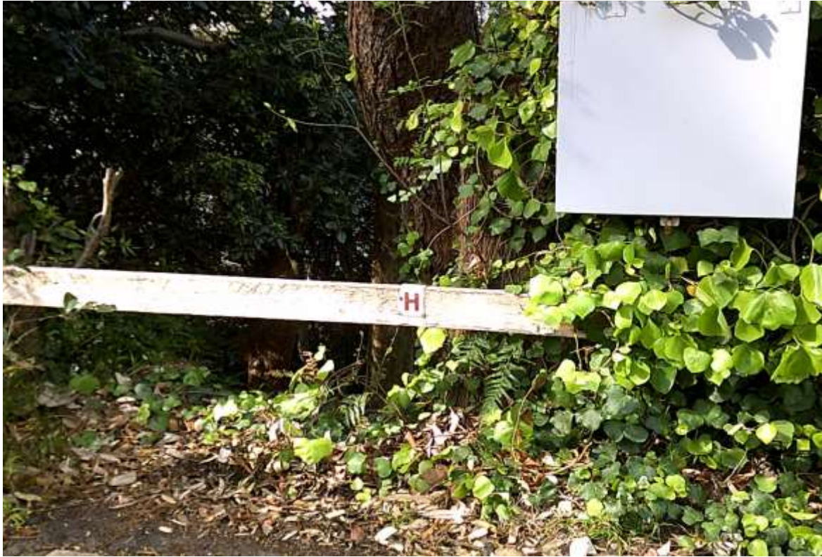
Photo 4 – Indicates the location of the nearest reticulated mains pressure fire hydrant adjacent to No.46 Beatty St at the end of the cul-de-sac (Steve Brooks 2020)
