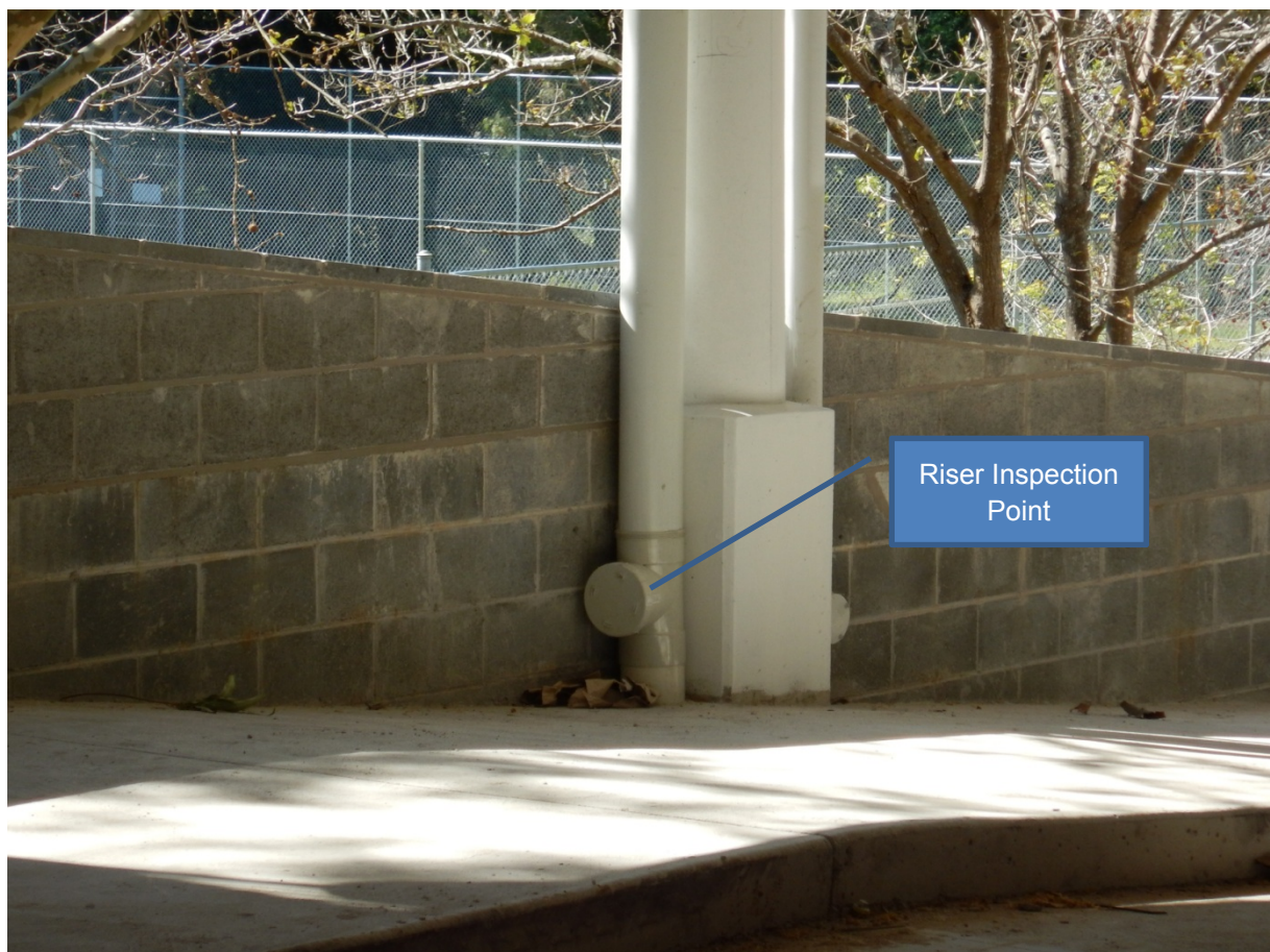
Photograph 1: Example of Riser Inspection Point
