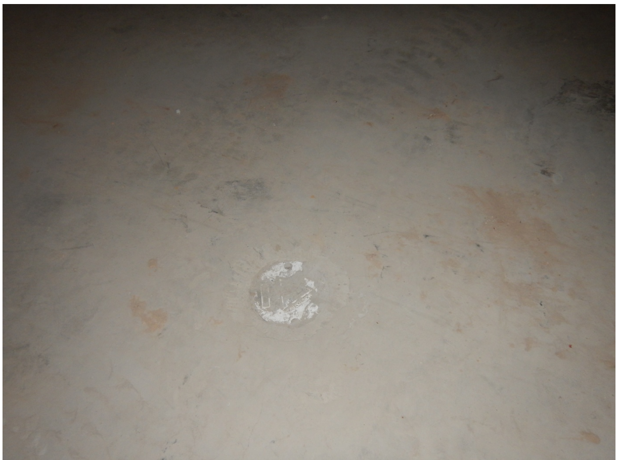
Photograph 2: Gravel Bed Inspection Point
