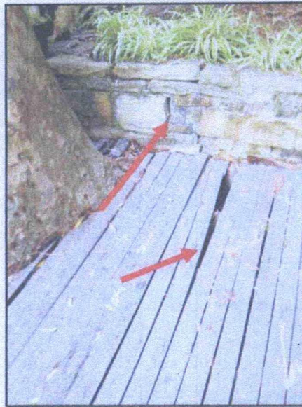
Photo 2: Damage to deck and retaining wall.
