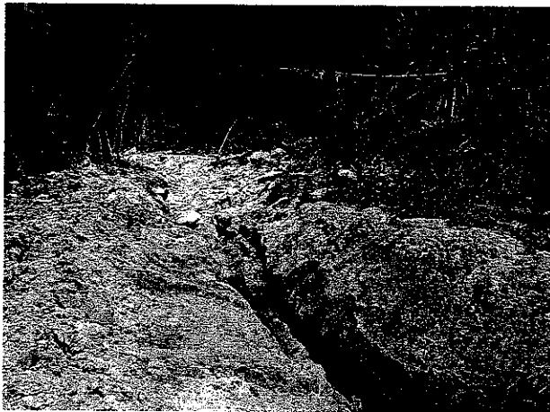
Plate13. Stormwater drainage ditch leading to wet/dry pond area.
