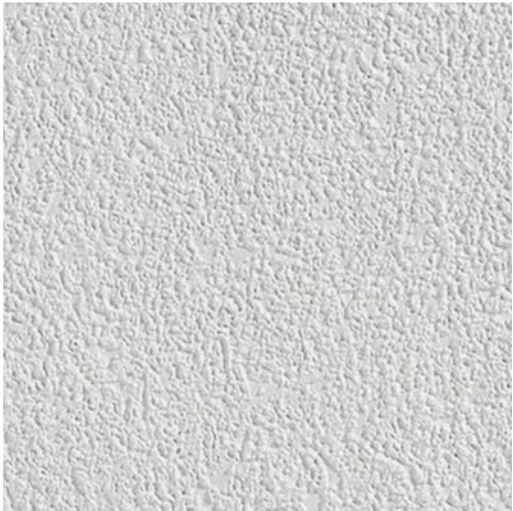
Rendered Masonry - lower level of existing dwelling - paint finish
