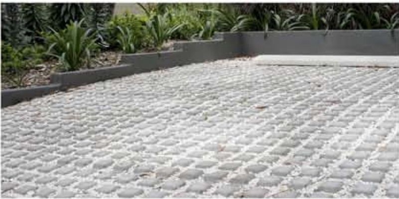
Permeable paving to portion of landscaping between carport and pergola
