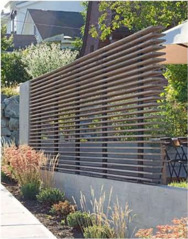
Timber and masonry boundary fence. 30% open above 1m.
