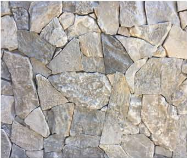
Stone cladding to external fireplace, BBQ rangehood and base of new fencing.
