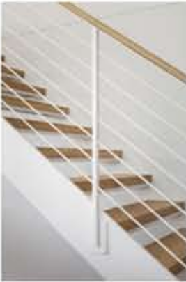
Timber treads and white powdercoated external stairs
