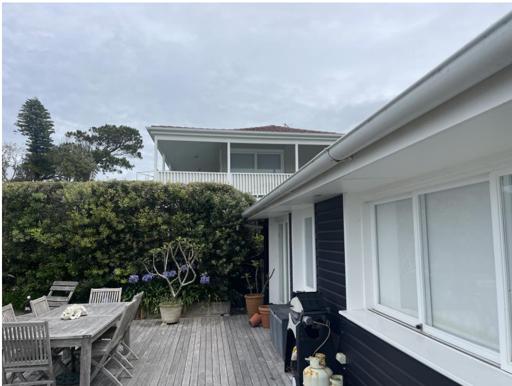
Fig 12: View looking south along the rear elevation of the existing dwelling, towards the neighbouring attached dwelling at No 87A Marine Parade
