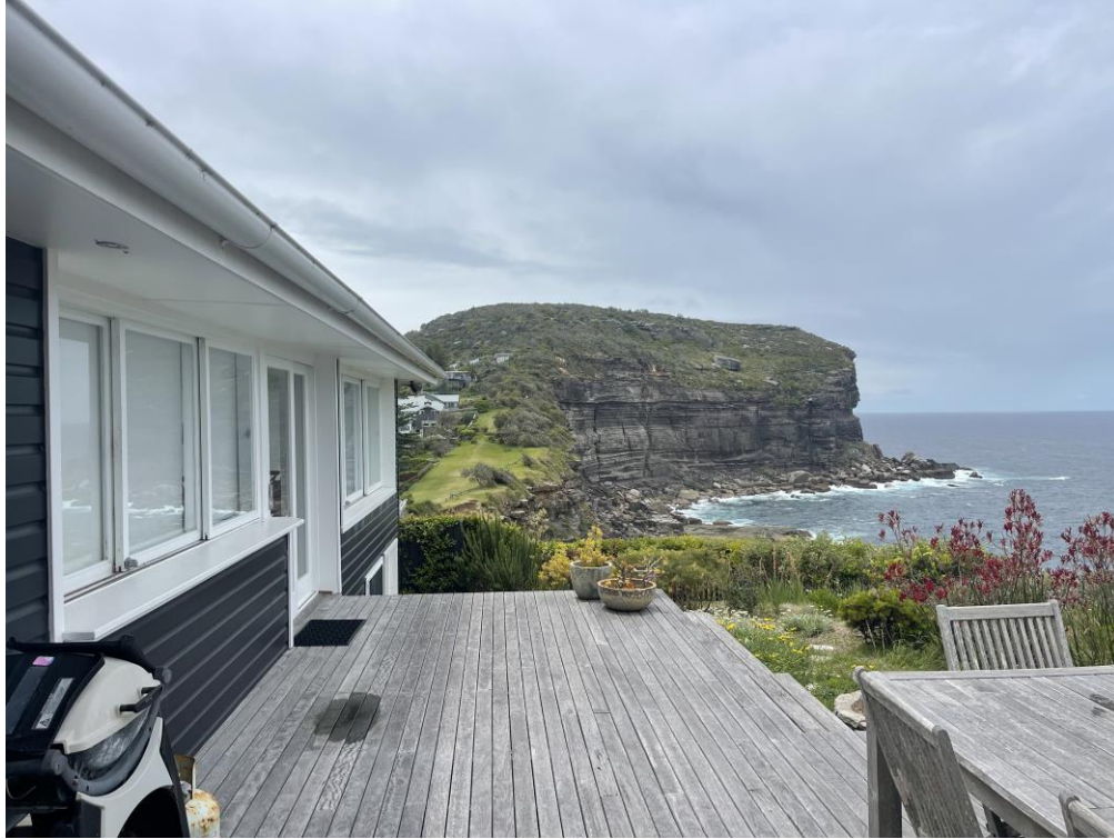
Fig 11: View looking north along the rear elevation of the existing dwelling
