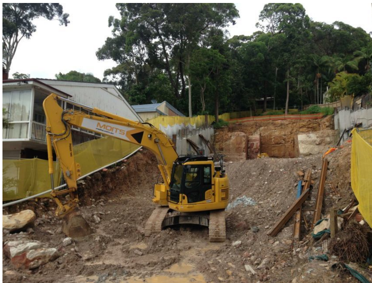
Photo: 1 – Development underway in No. 2079
