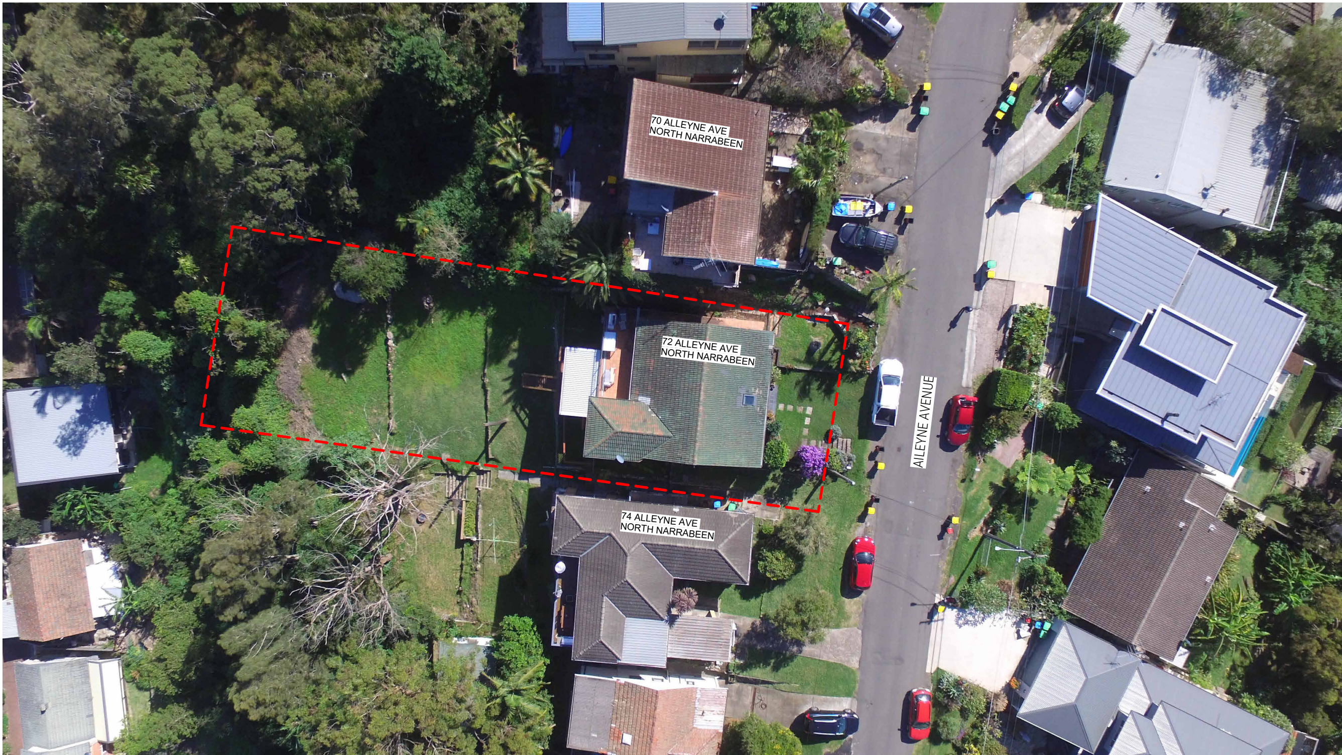
TOP OF ROOF DRONE VIEW
