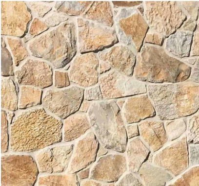
YELLOW SANDSTONE CLADDING FOR RETAINING WALL
