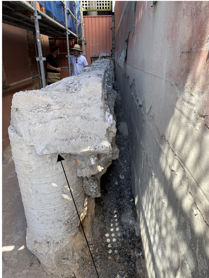
Piles to be trimmed
