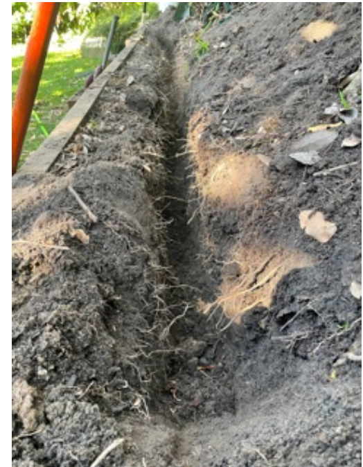
Image of trench East to West
