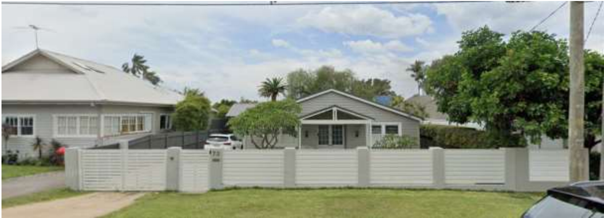
View of Subject Site from Hay Street
