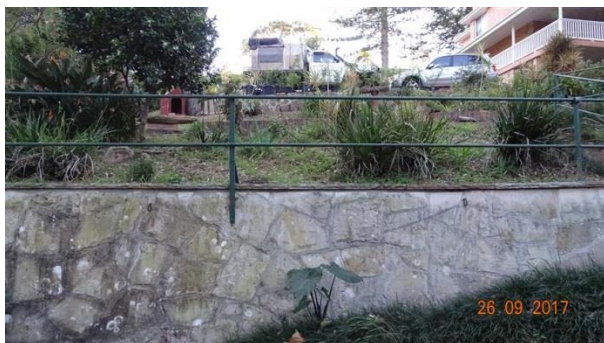
Western Side of Property Above Retaining Wall
