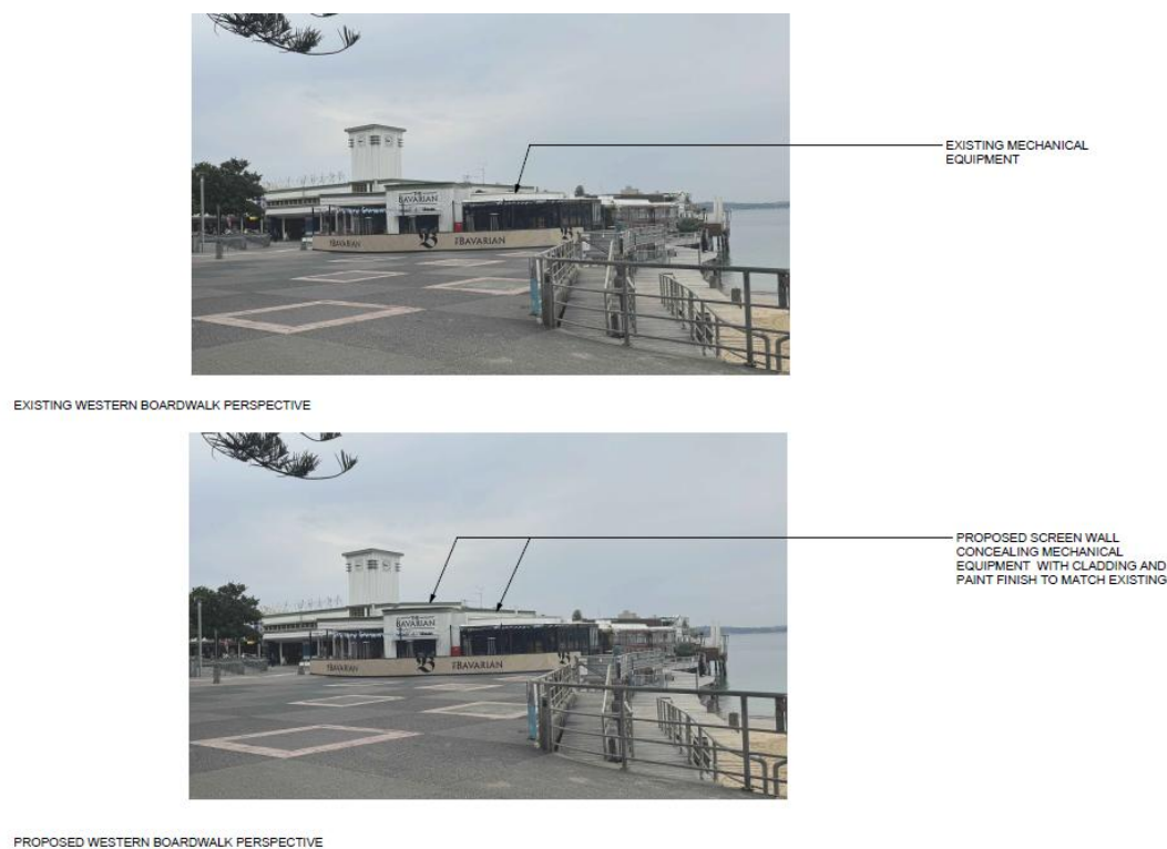
Figure 13: Western elevation perspective showing existing mechanical equipment above the roof of Manly Wharf, and the proposed screen wall to conceal this equipment. Source: Little Boat Projects, Drawing No. D.03.153, rev. DA1.
