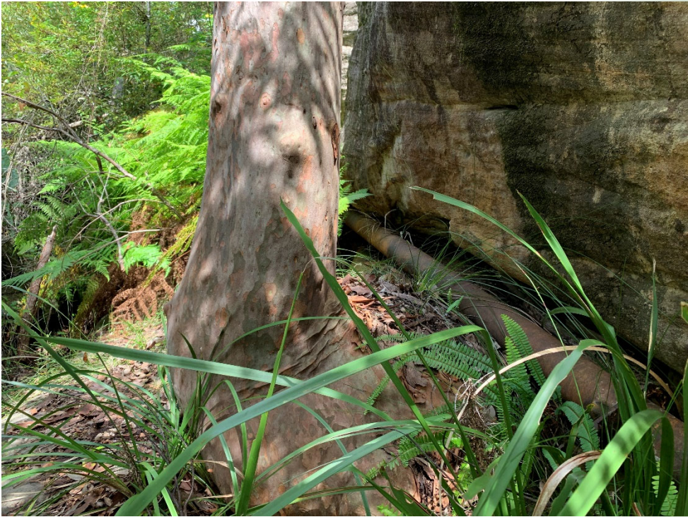
Figure 4.3 - The base of Tree No. 96.1 showing the existing cast iron rising sewer main.
