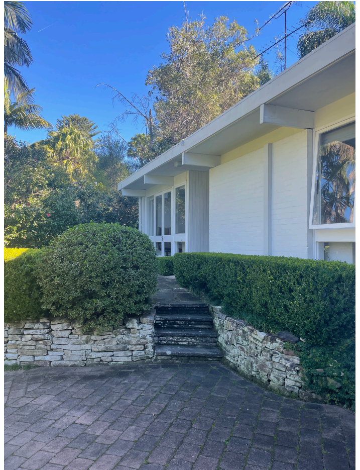
View of the front of the house which features an expressed timber frame and wide eaves and exposed rafters. The landscaping incorporates dry stone walls.
