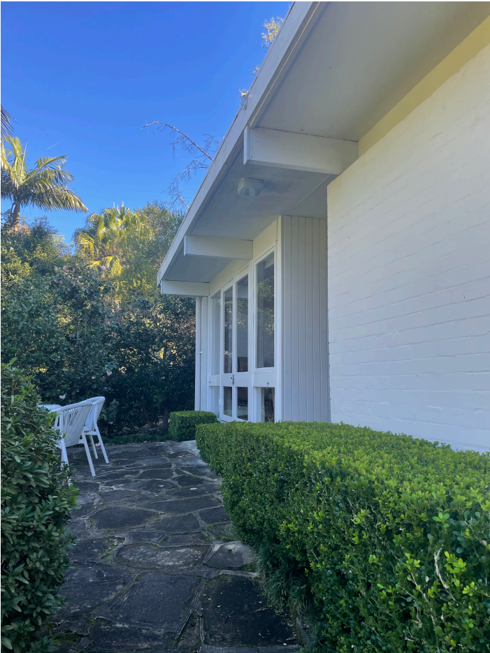
View of the front terrace of the house. The timber framed doors are contained in a projecting bay.
