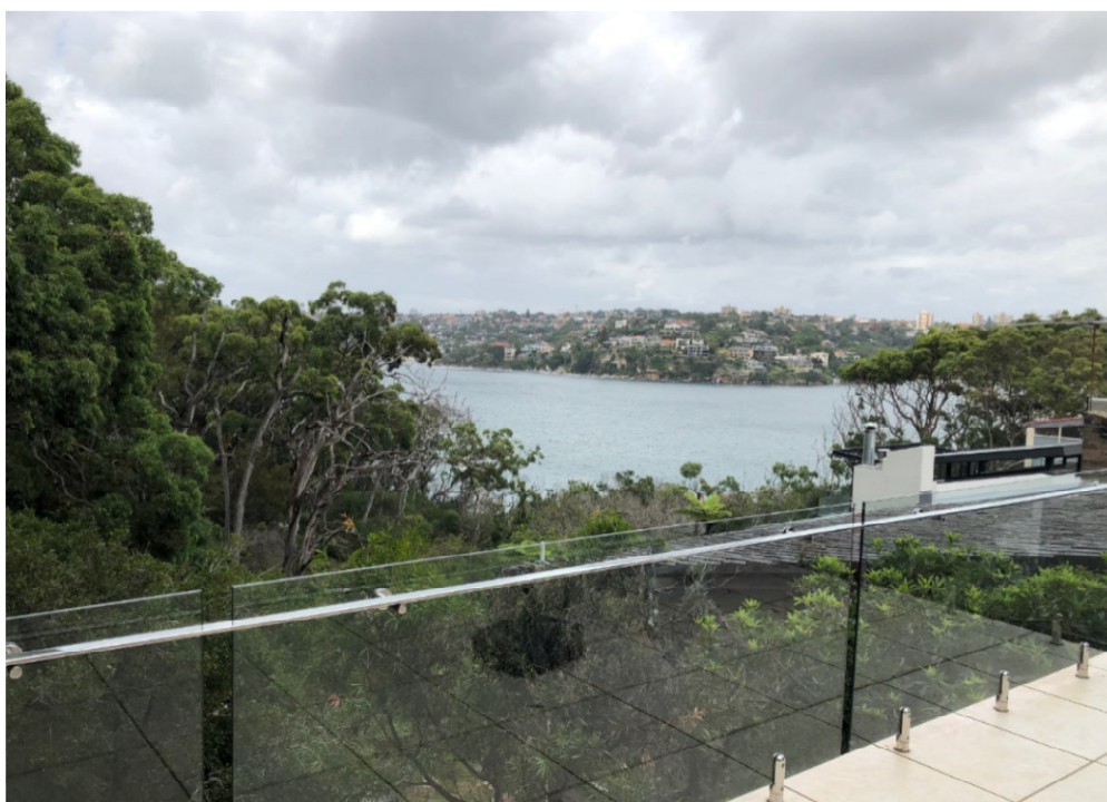
Photo 1- Ground floor terrace (standing)
