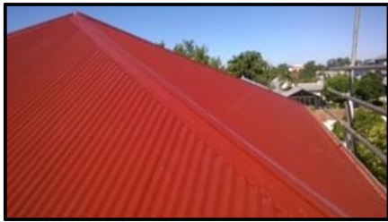
MT-01 COLOURBOND METAL ROOF SHEETING POWDERCOAT FINISH 'MANOR RED' OR SIMILAR WHERE MARKED ON ELEVATION.
