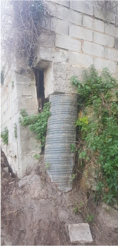
Photograph 9: View of the deformed pier at the corner of the site and outwash sand
