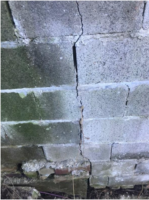
Photographs 6 and 7: Near vertical cracking in retaining wall taken from the southern side looking broadly north.
