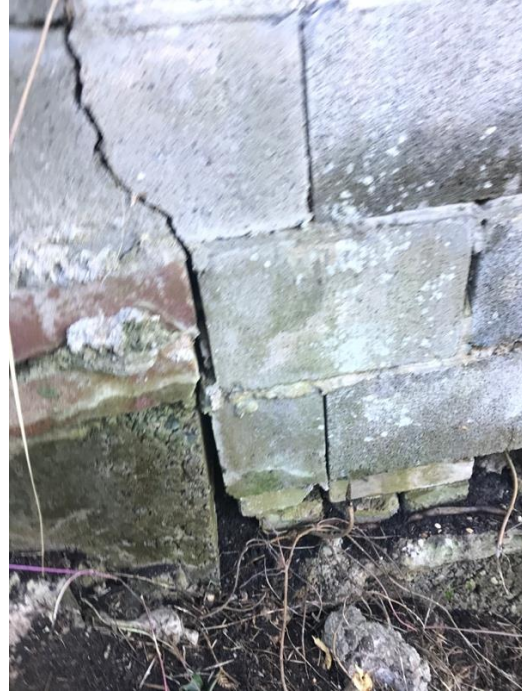
Photographs 6 and 7: Near vertical cracking in retaining wall taken from the southern side looking broadly north.
