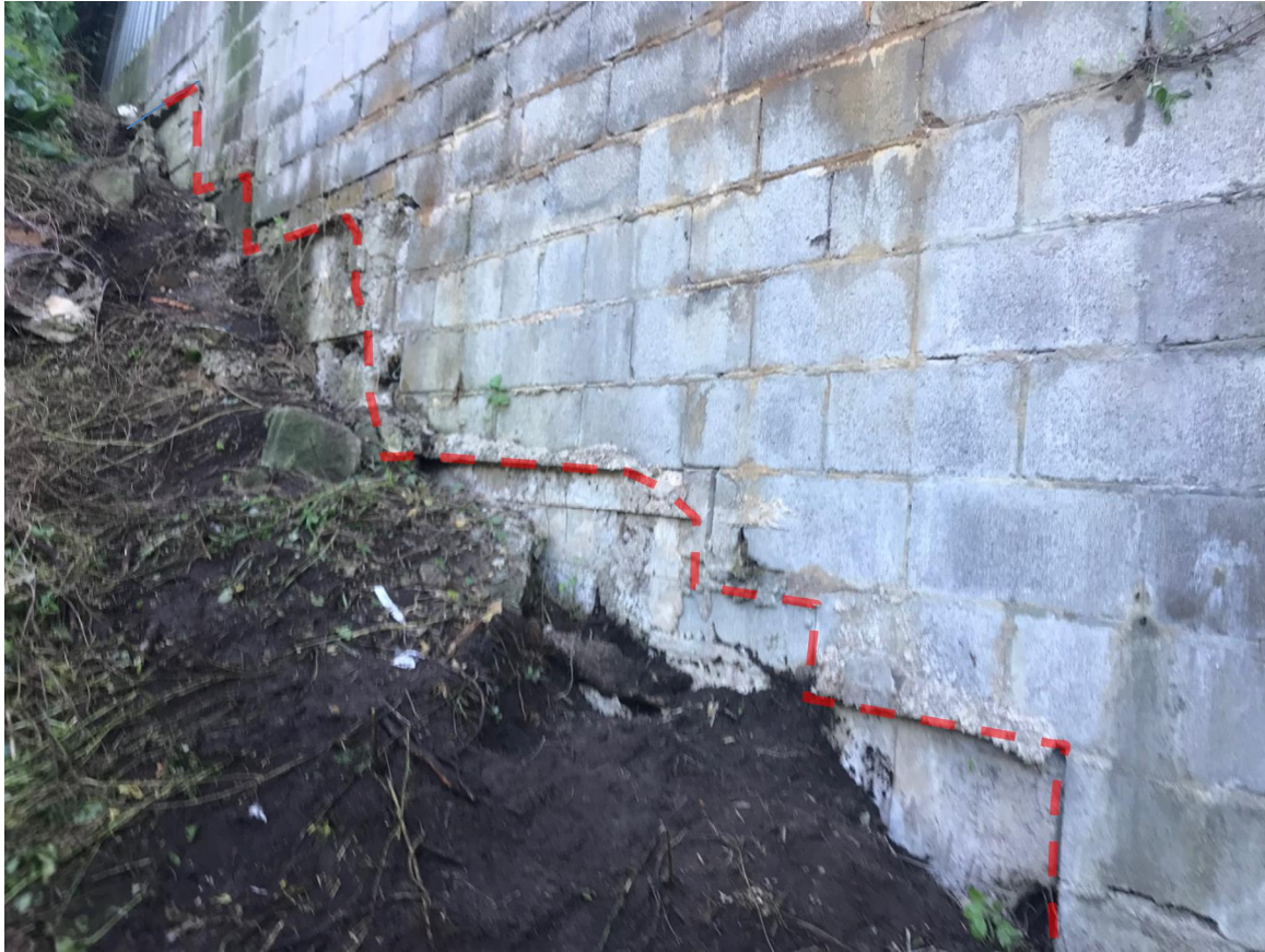
Photograph 8: Probable original ground line (dashed red) on south side of retaining looking broadly west from the east end of the wall.
