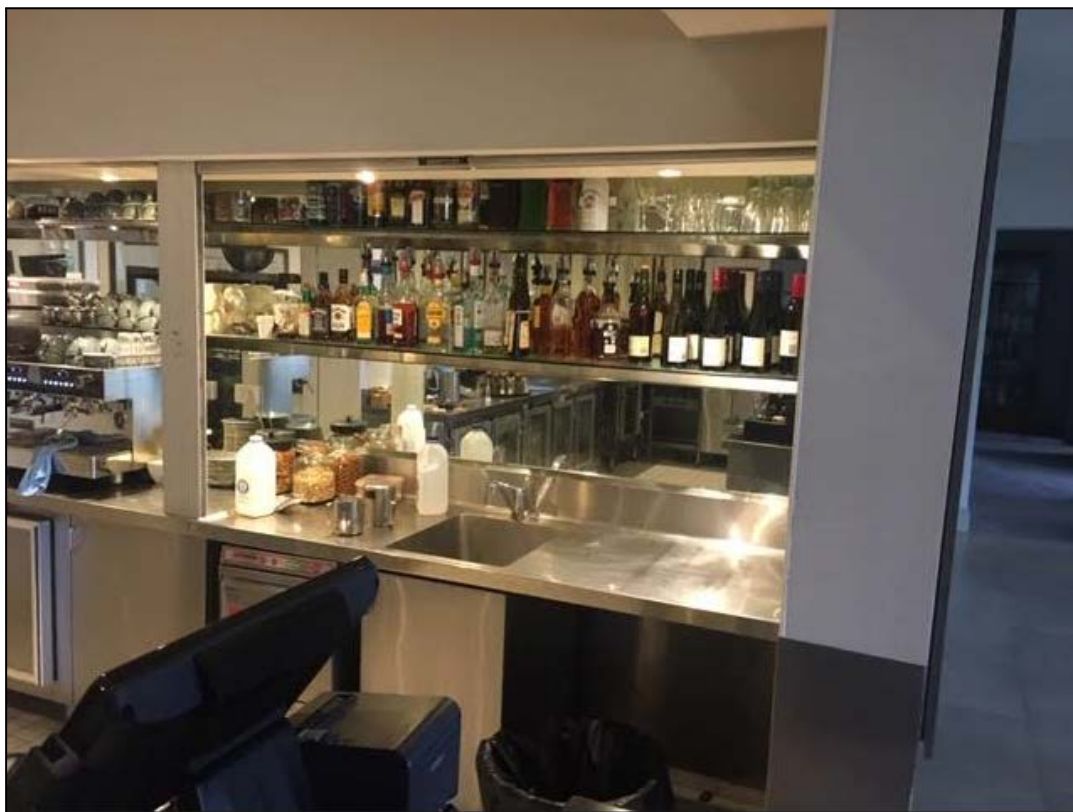
Figure 4: This section of bar including the wall will be removed. The wall is not structural.
