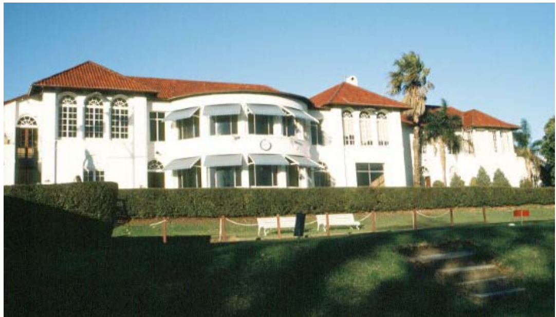
Figure 17: The subject site in the 1986 heritage study. (Source: NSW Office of Environment and Heritage database)
