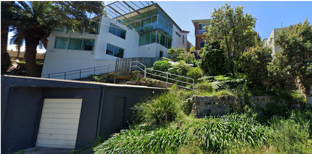
View Site from Aitken Avenue
