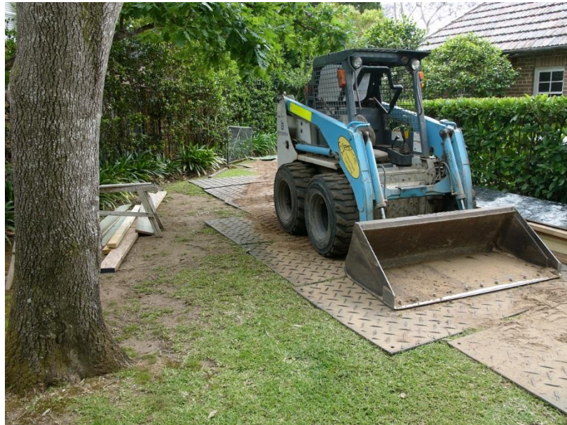
Figure 4 – Showing typical detail for truck mats.
