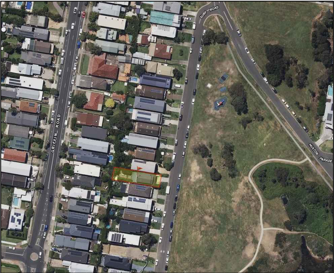
Areal View with Highlighted the Location of the Residence at No.30 Surf Road, NORTH CURL CURL
