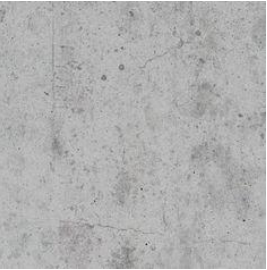
OFF FORM CONCRETE PRECAST WALL PANEL
