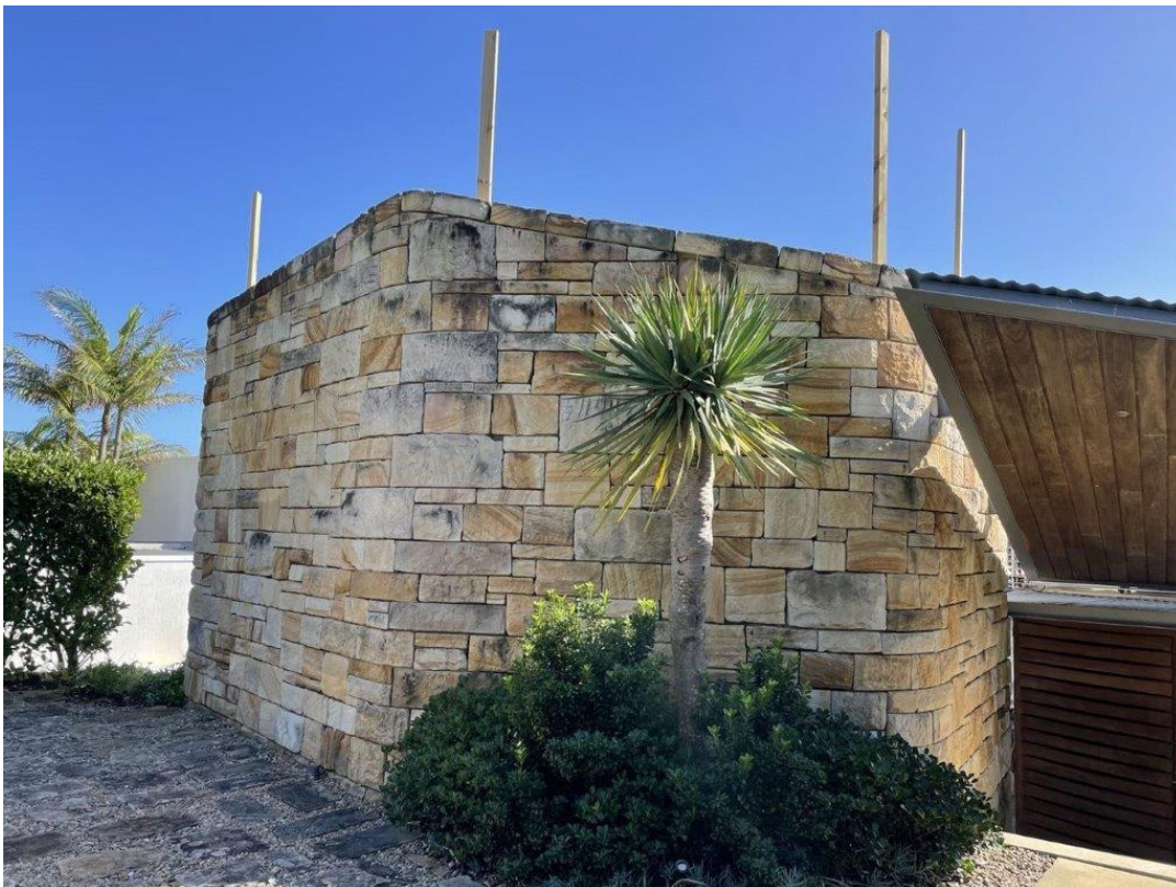
Figure 5 – existing stone clad structure and dwelling entry to the south
