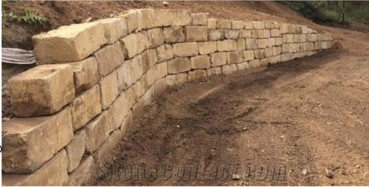
→ Sandstone retaining wall
