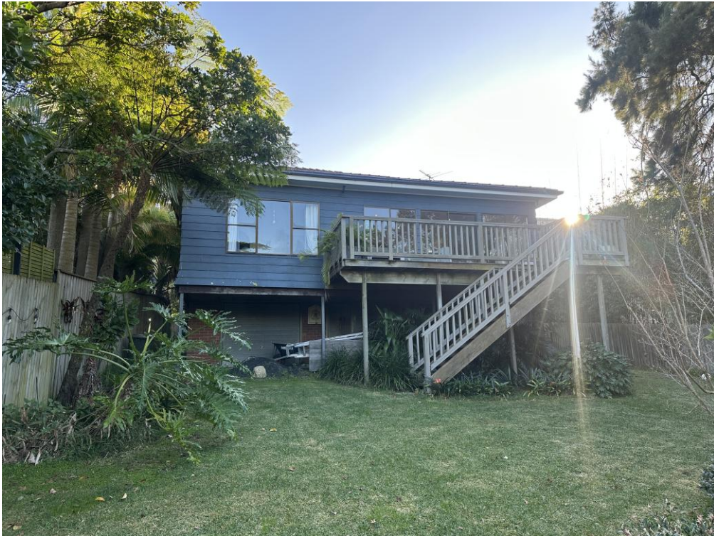
Figure 8. The existing deck and rear landscaping to be reconfigured under this proposal
