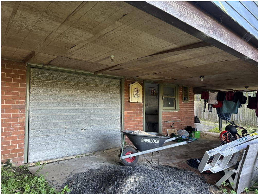
Figure 9. Existing undercroft to be reconfigured under this proposal
