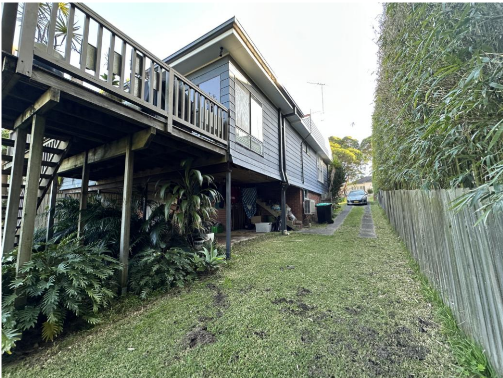
Figure 7. eastern side of the existing dwelling viewed from the rear of the site
