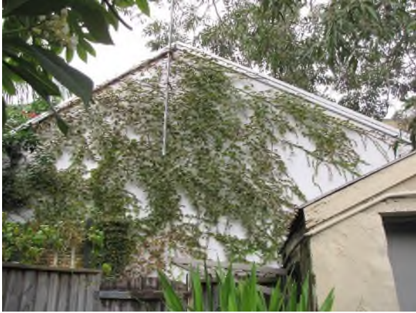
Figure 15: End wall of No 26 Denison Street.
