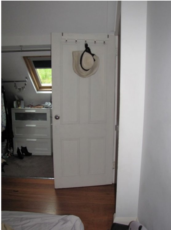
Figure 23: Attic room – original door & wide floorboards, later joinery and plasterboard linings.
