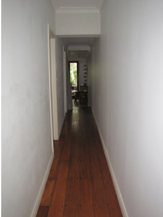
Figure 21: Hallway with original flooring, later skirtings, architrave and cornice.
