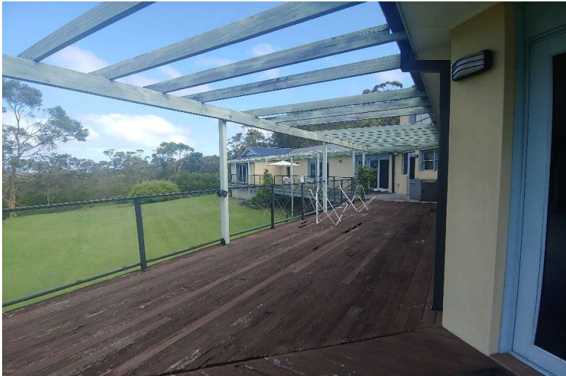
Above: Existing deck viewed from the north
