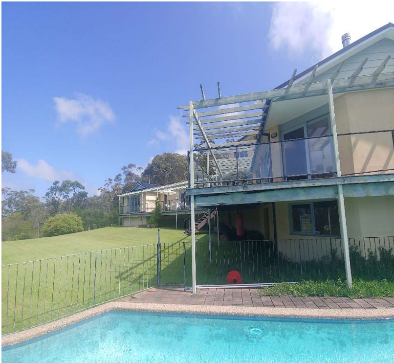
Above: Existing pool area and deck viewed from the north
