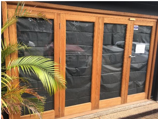
Figure 5.3.8a – Main entrance door
