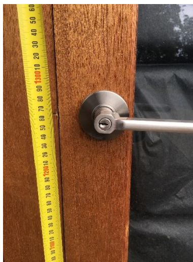
Figure 5.3.9 – Height of operative latch
