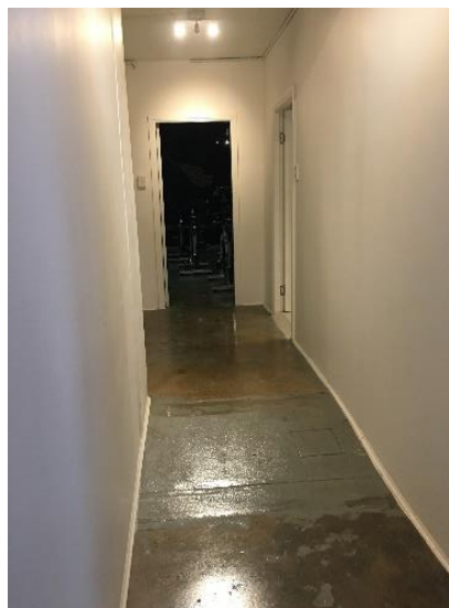
Figure 5.2.2 – Internal walls and ceilings in the corridor
