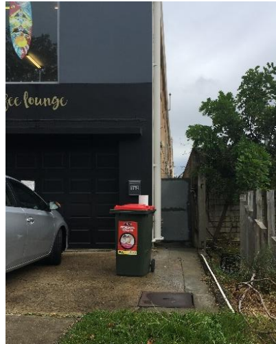
Figure 5.2.3a – Opening along the eastern elevation
