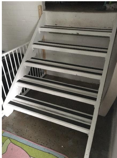
Figure 5.3.7 – Stairway serving the storage area
