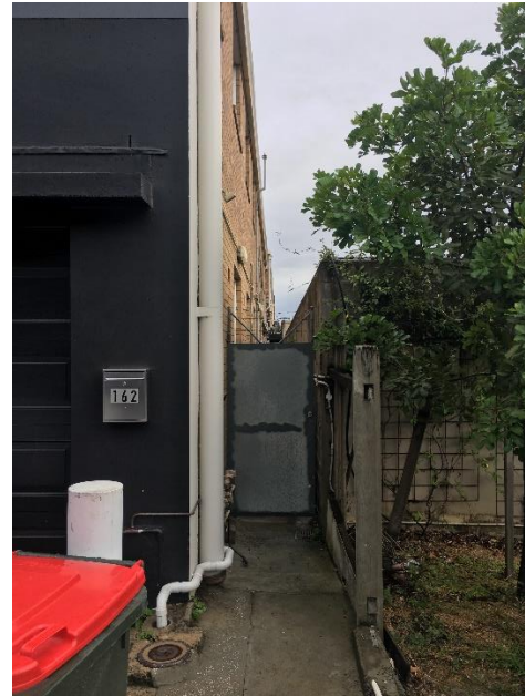
Figure 5.2.3d – view of external wall along northern boundary
