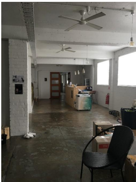
Figure 5.4.5c – No directional exit signage
