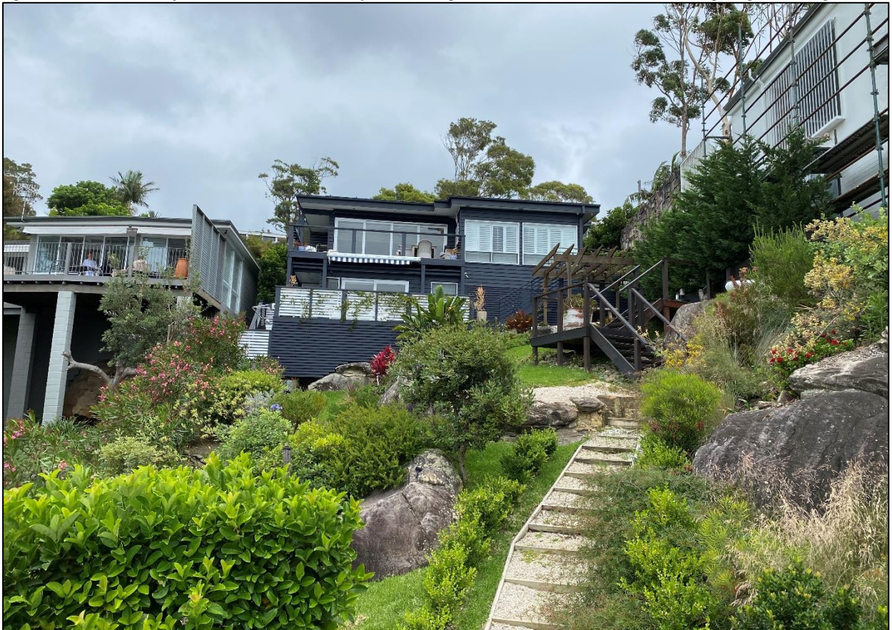
Figure 8. View from subject site lower end of rear yard showing cross fall of site and relative building heights to neighbour
