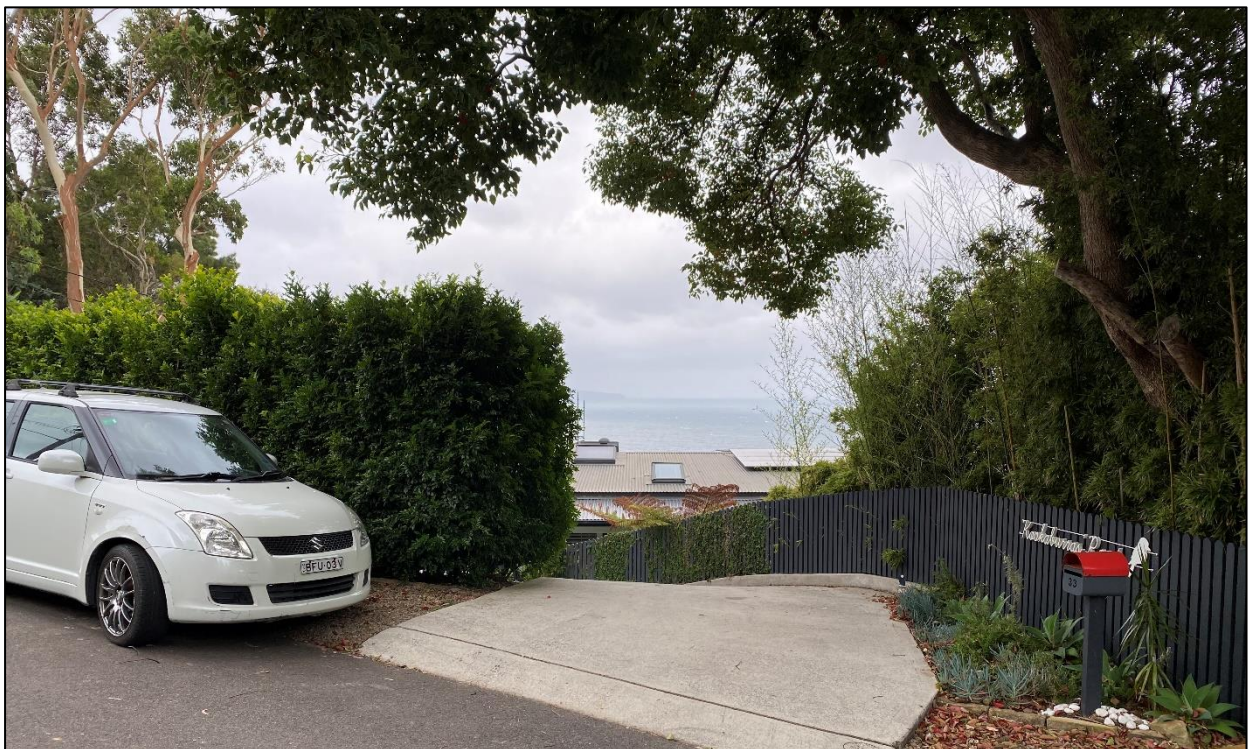
Figure 2. View of existing dwelling from Pacific Road through the driveway from SW
