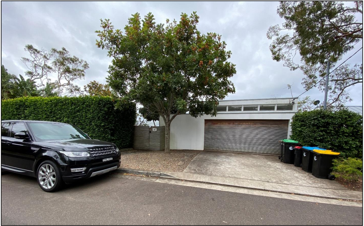
Figure 9. View of 41 Pacific Road with NIL front setback to garage and landscape screen to road reserve
