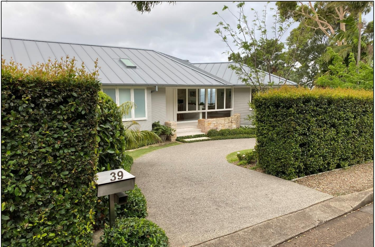
Figure 10. View of 39 Pacific Road with landscape screen in road reserve and front setback reduced
