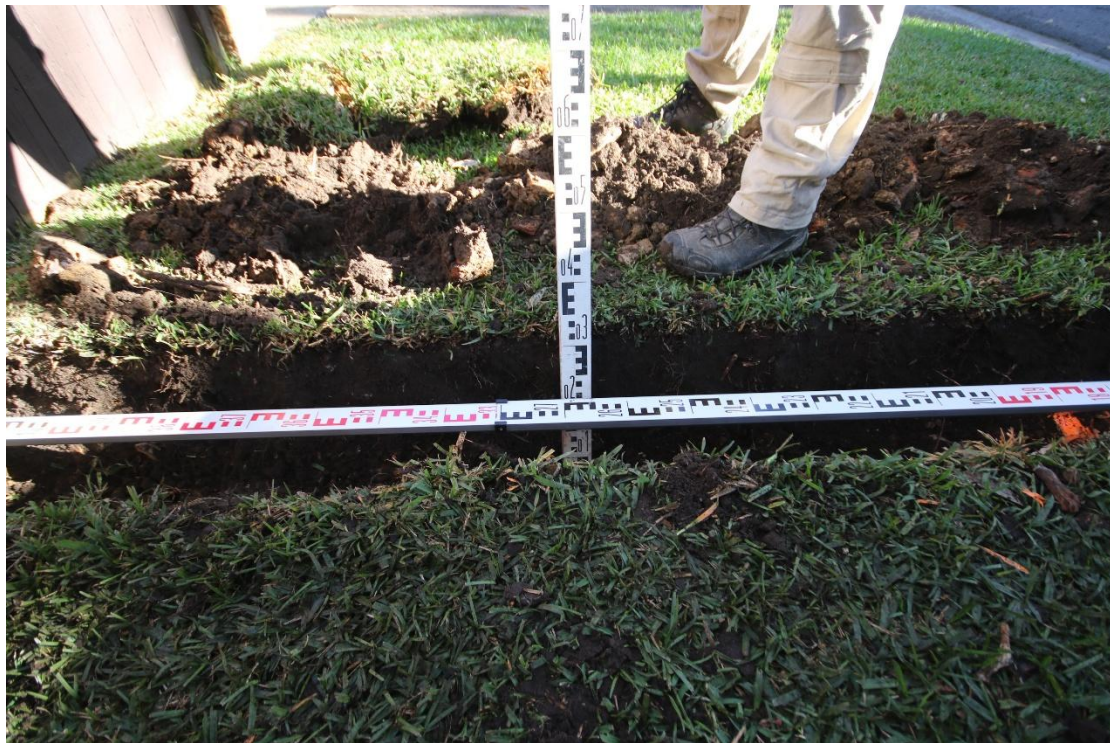
Plate 20: Trench 2 depth of 350mm at 2.65m from behind the kerb.
