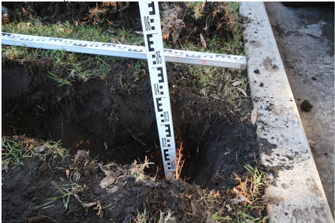
Plate 17: depth of trench 1 behind the kerb.
