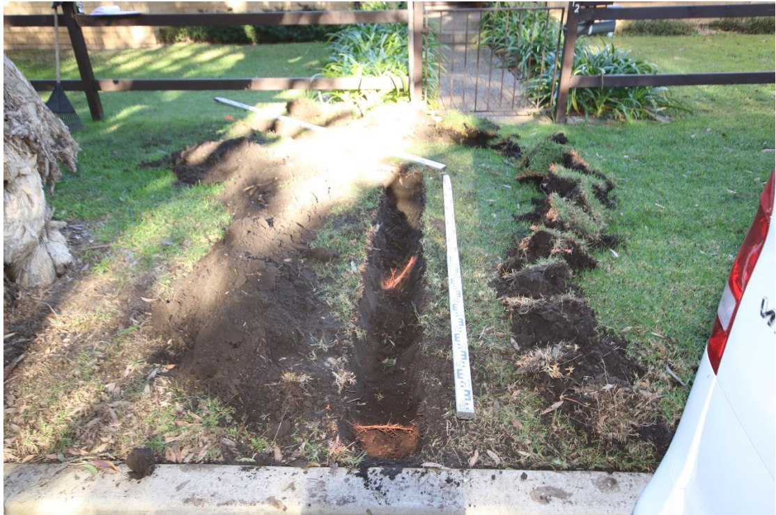
Plate 13: Overall view of trench 1.
