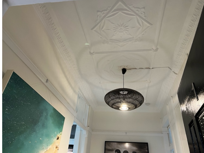
1/18 Quinton Rd – Entry corridor - Example of ceiling details
