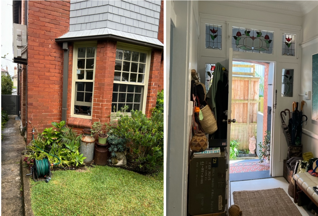
View of Timber Windows and Doors to 1/18 Quinton Road
