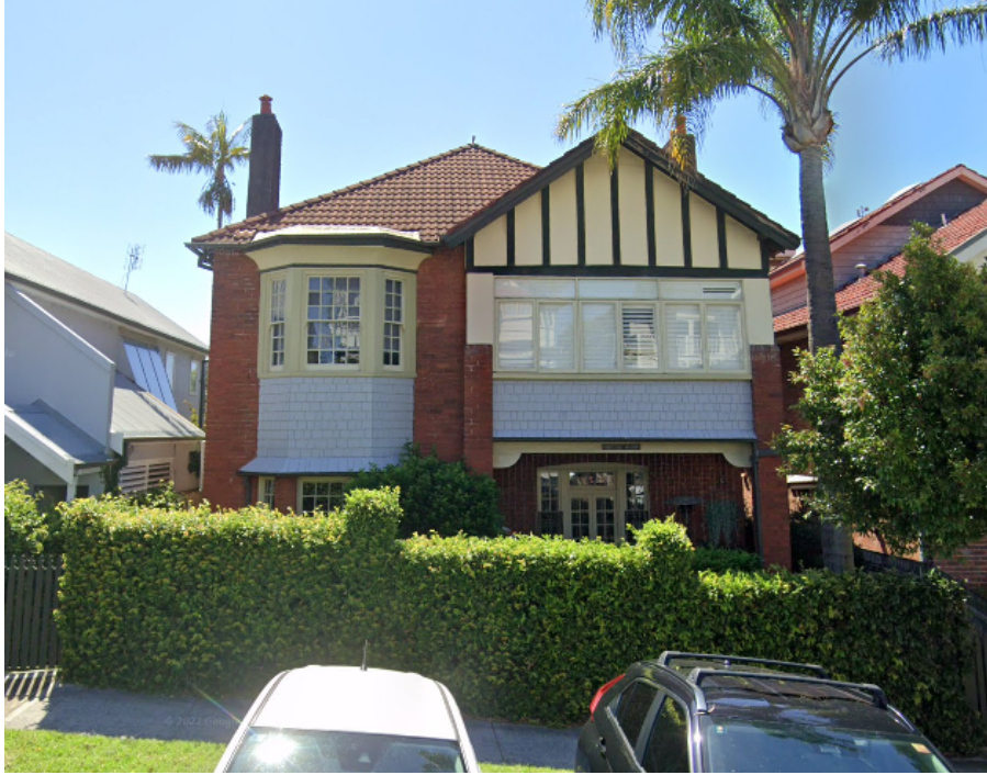
18 Quinton Road – As viewed from street level
