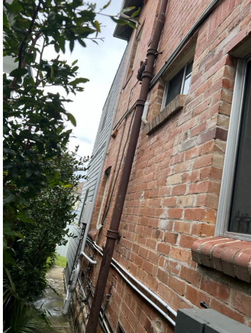
View of Junction between 18 and 22 Quinton Road
