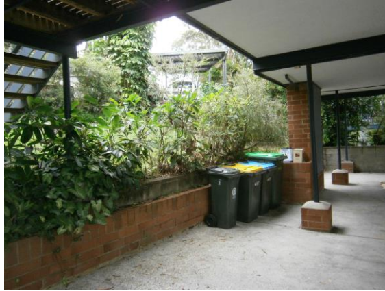
View looking south east up towards the street. Lower ground area to be enclosed
