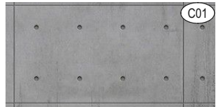
OFF FORM CONCRETE
