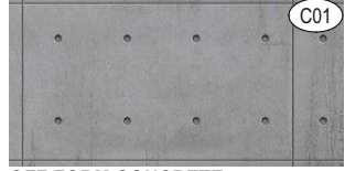
OFF FORM CONCRETE
