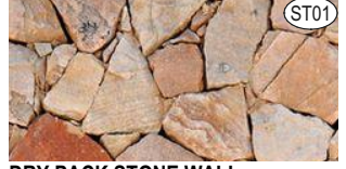
DRY PACK STONE WALL
