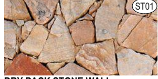
DRY PACK STONE WALL
