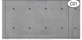
OFF FORM CONCRETE
