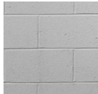
1. Existing Concrete Block Wall Colour: White
