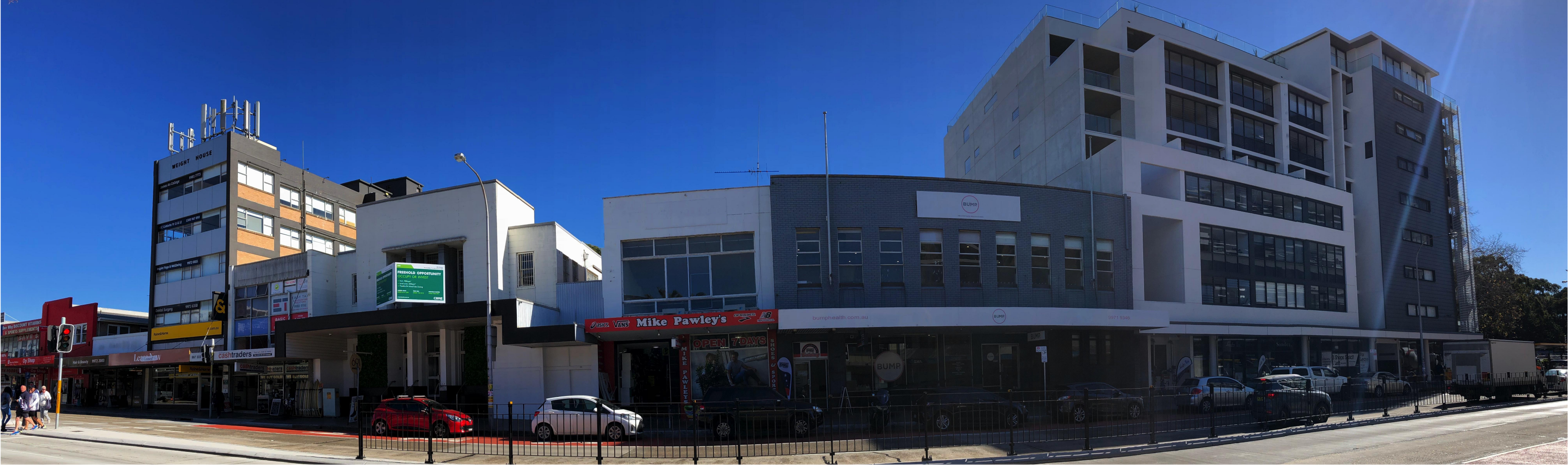
EXISTING SITE PANORAMIC PHOTO
