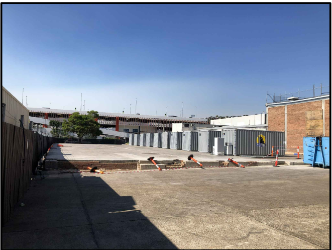
9. FROM SITE LOOKING SOUTH
