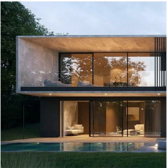
FEATURE WALL - OFF-FORM CONCRETE
