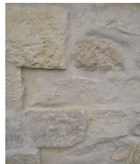
LIME WASHED STONE
