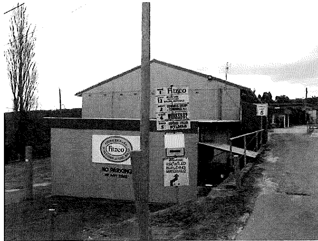
The westernmost building (to be demolished)
