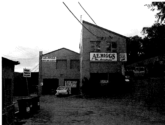
Existing building proposed for partial retention
