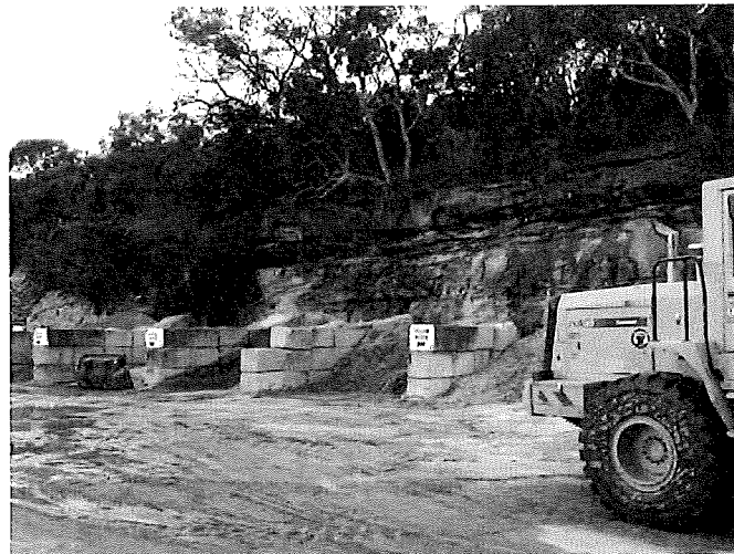
Storage of sand and soil
