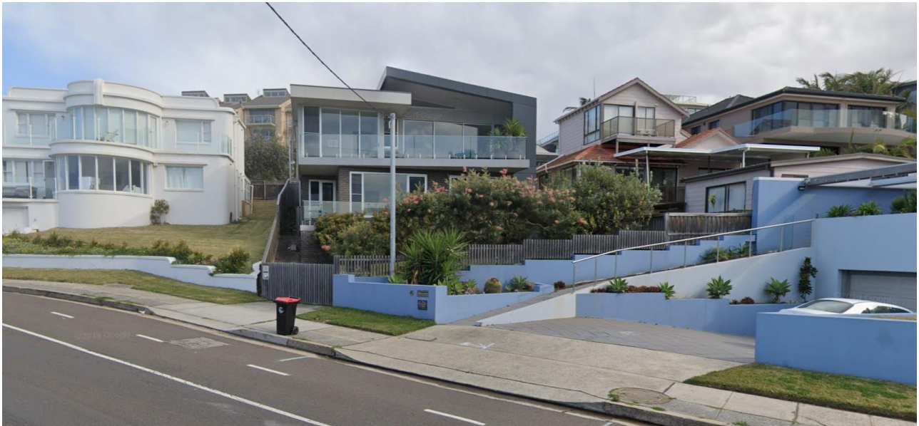
The view of the existing house from Carrington Parade.
