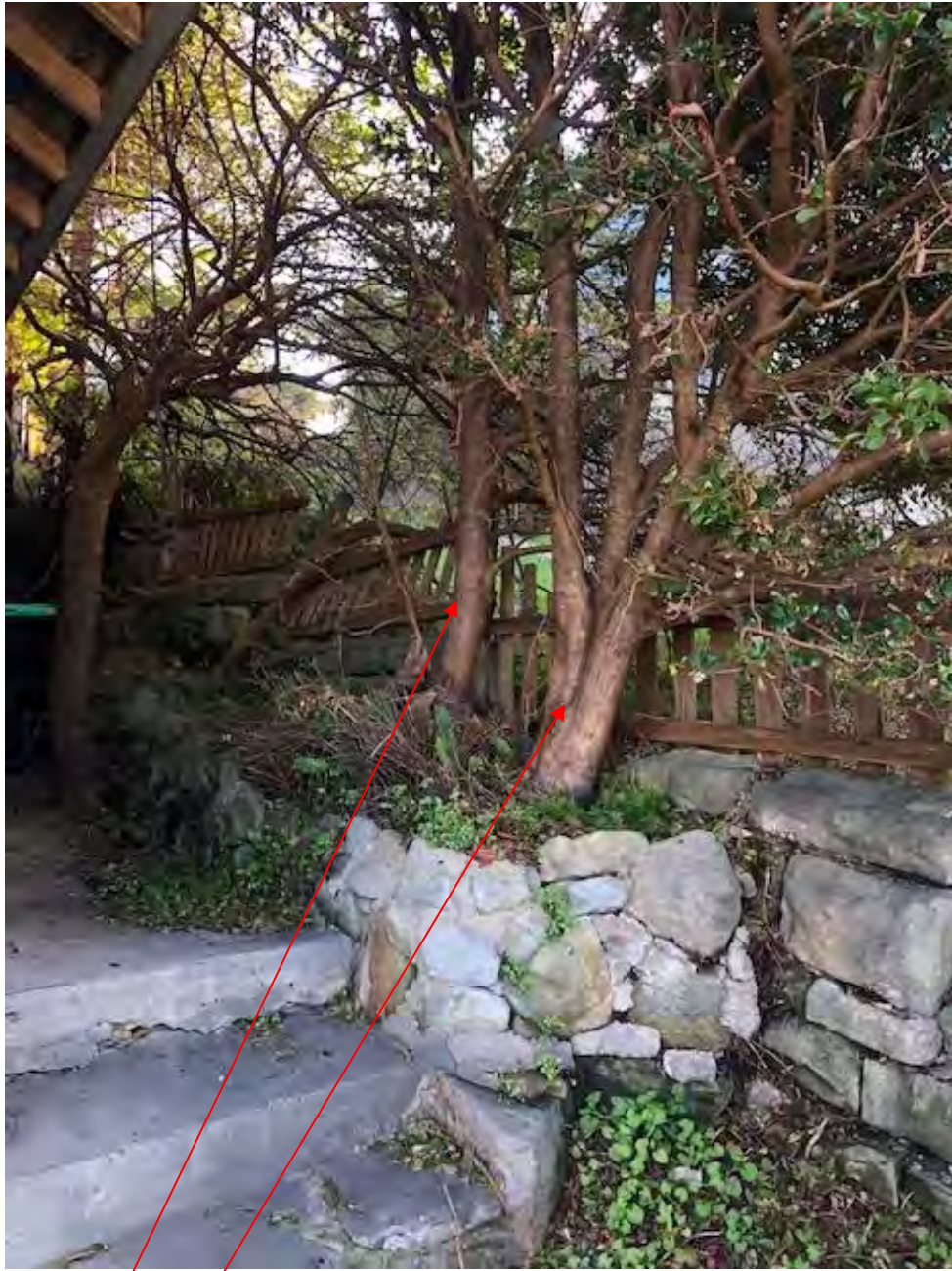
Photo B: Trees 6 and 7 within 2 metres of the existing dwelling.
