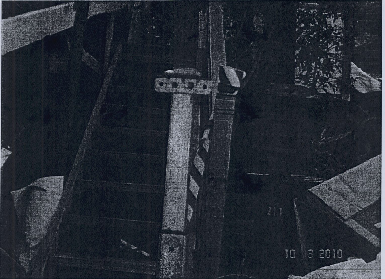
PHOTO 42: Temporary site stairs.
