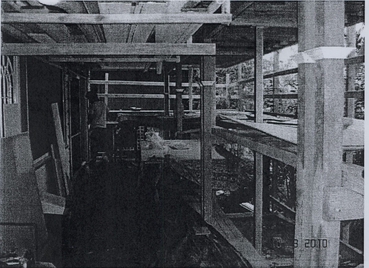
PHOTO 32: Decks being extended.
