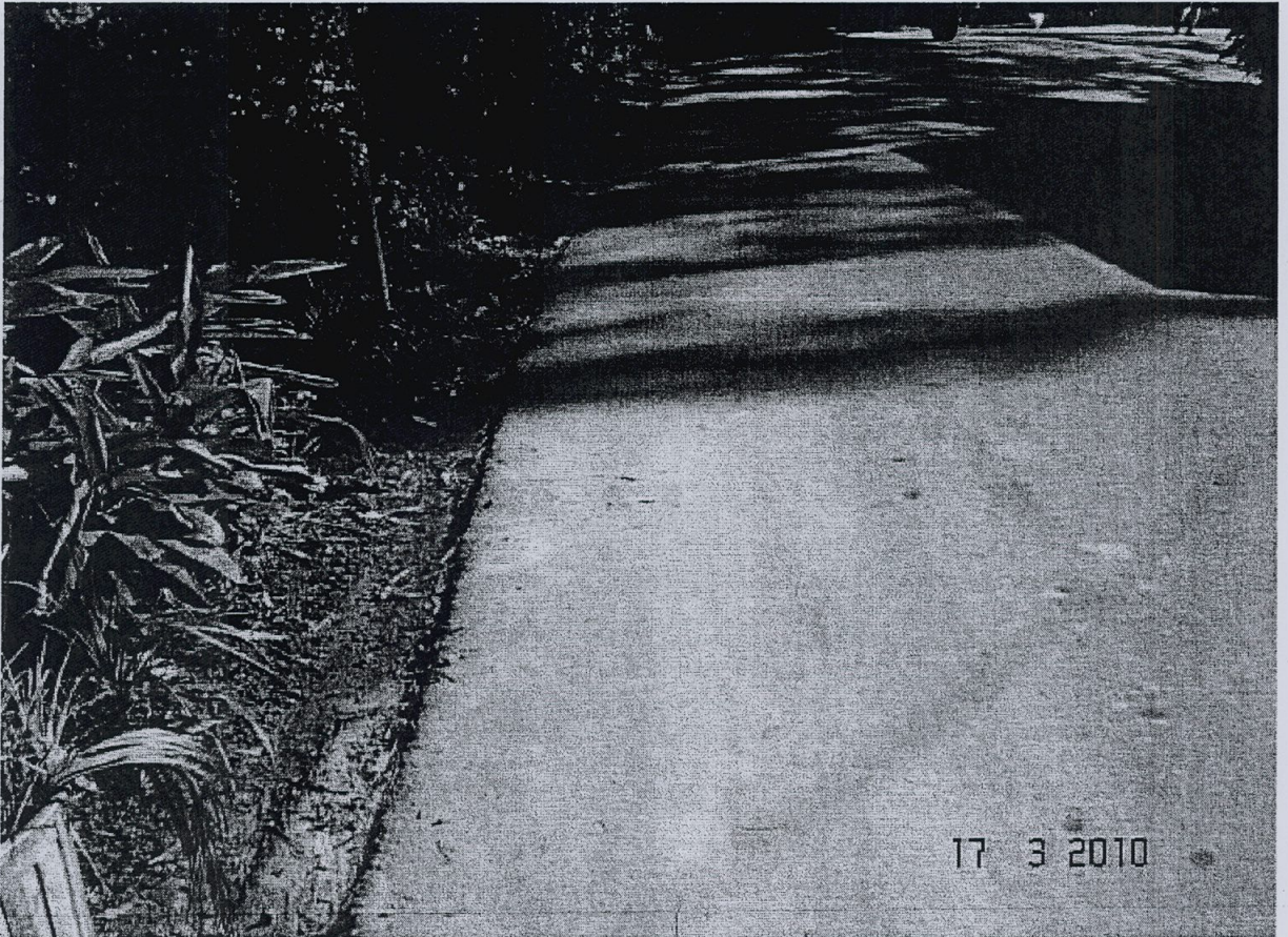
PHOTO 3: Previous cracking not evident.
